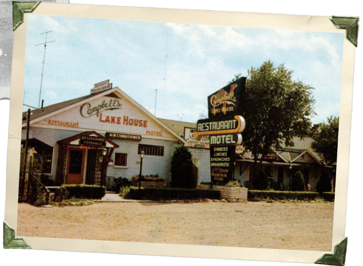
Built in 1946, Campbell's Lake House motel was expanded in the 1960's. The second story addition and more square footage provided space for a restaurant.
