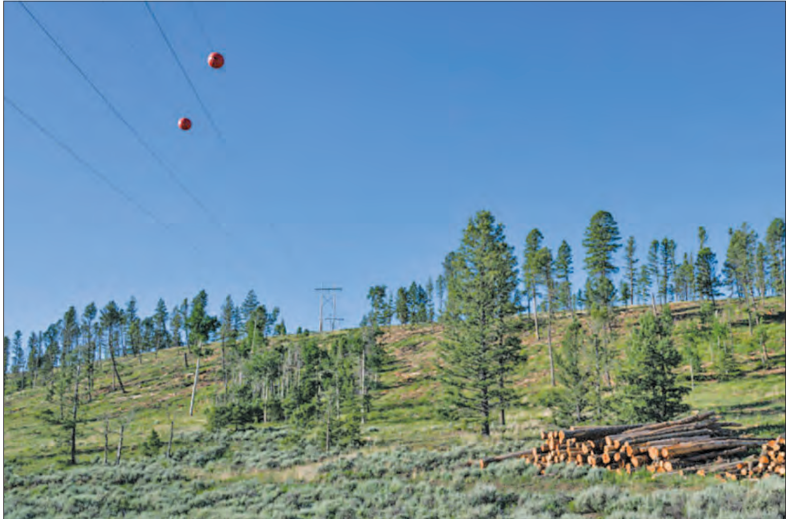
Power lines over Poncha Pass serve the San Luis Valley. According to the Colorado State Forest Service, Western Spruce budworm and Douglas-fir beetle have decimated trees in the area. The dead and dry timber has increased fire risk in the area, which may imperil the power lines.
