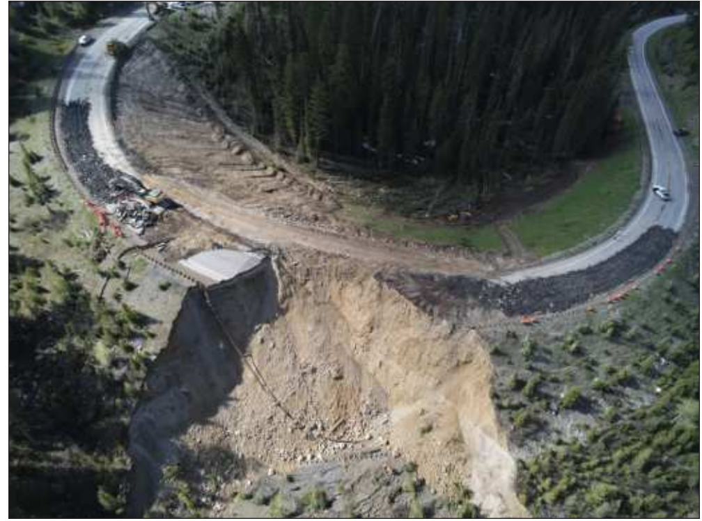
Photo courtesy of Wyoming Department of Transportation
