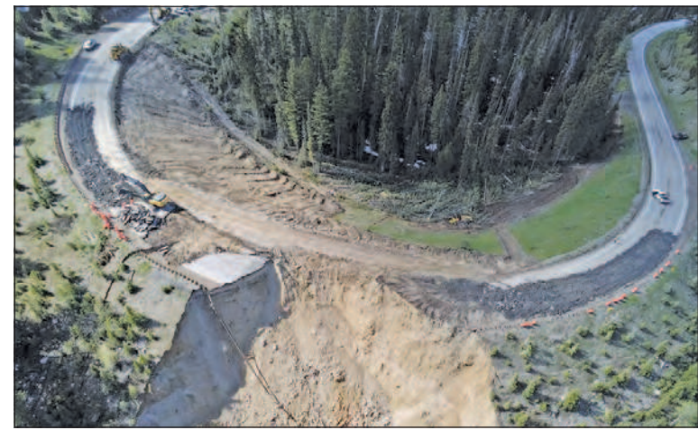
Photo courtesy of Wyoming Department of Transportation
