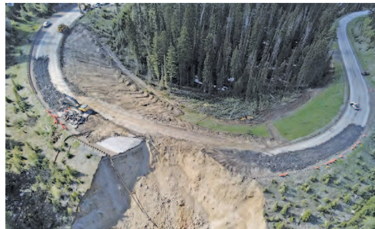
Photo courtesy of Wyoming Department of Transportation
