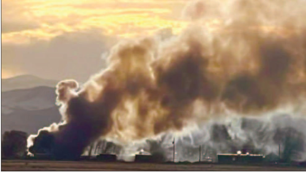
Courtesy of Saguache County Emergency Management Facebook page Saguache County Sheriff Dan Warwick said fire continued to burn inside the walls of a Moffat home and plans called for bringing in an excavator to bring the structure down to continue fire suppression.
