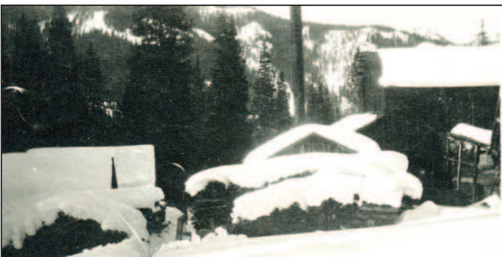
Buildings at the Sulfur Mine southwest of Creede during a very snowy winter around 1925. This photograph was made into a postcard. John LaFont Collection, Creede Historical Society Archives, Catalogue #5179-JLF-75.
