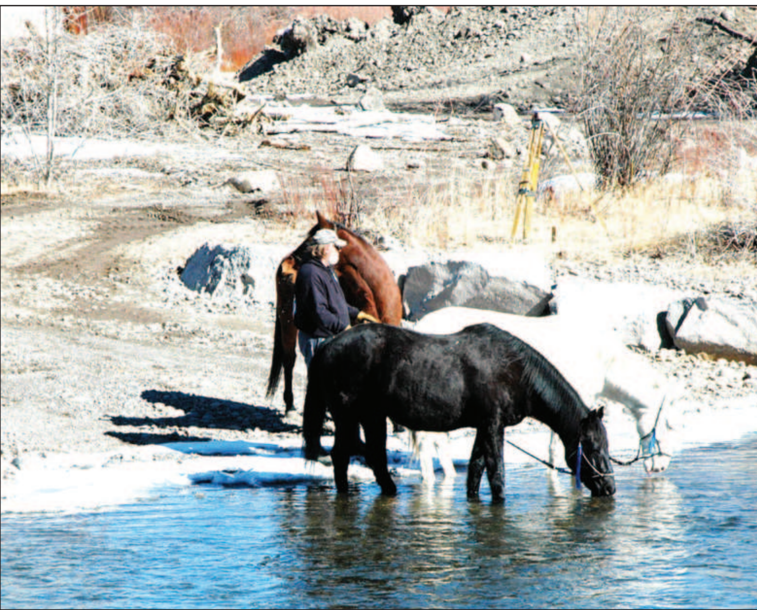
Del Norte Riverfront Project Construction's new boat ramp services diverse user groups. "We took (a photo) looking across the Rio Grande today while standing on the fishing pier — a surprise user group — no one had thought of horses using the boat ramp," said Bonnie Asplin, from the Del Norte Trails Organization. "We thought it was great!"
