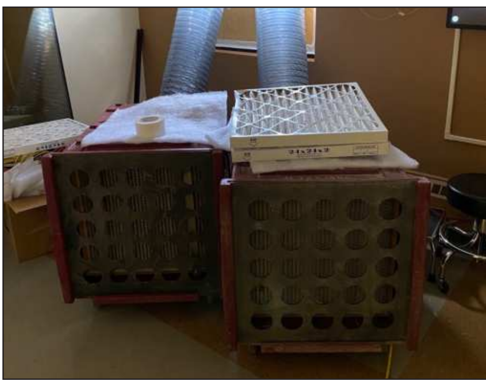
Photo courtesy of SLV Health Negative Pressure Ventilation at Stuart Avenue Respiratory Clinic
