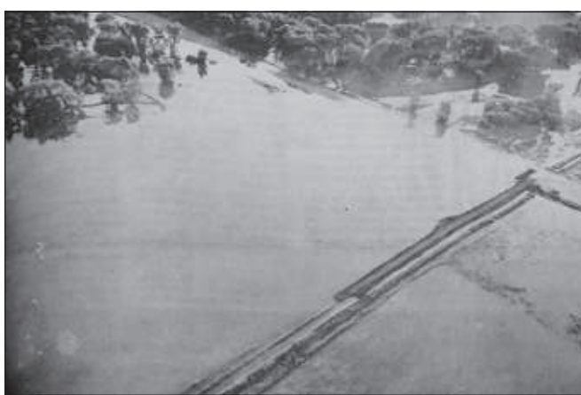
Monte Vista Journal, June 12, 1985 Below: The banks of the Rio Grande river are obliterated in this aerial photograph. In the right background, dirt lines the bank to help stem the flow while (right, center) police vehicles are grouped to enforce the "no through traffic" policy enacted for a portion of Hwy 285.
