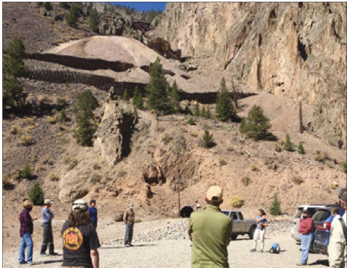
Folks meet at the Nelson Tunnel to talk about historic structures, Fall 2020.
