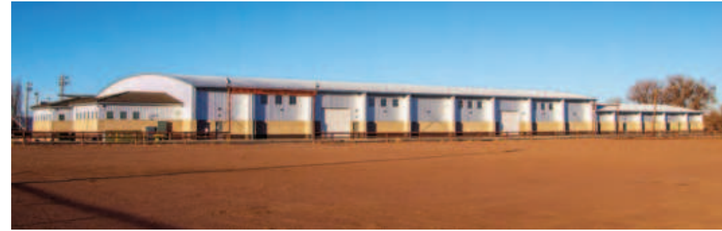
Completed building at a glance — Page 5
