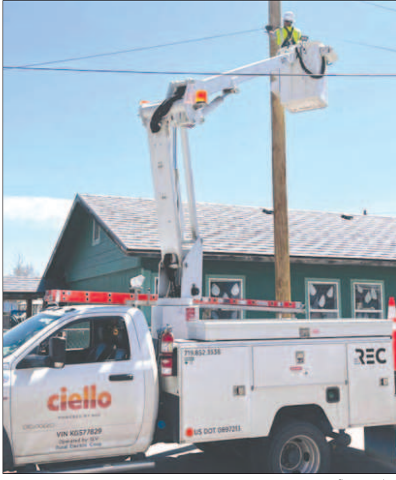
Courtesy photo An SLVREC/Ciello lineman is shown installing fiber optics at an SLV home.
