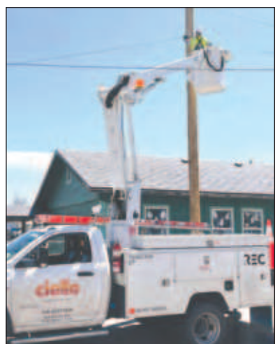
Courtesy photo An SLVREC/Ciello lineman is shown installing fiber optics at an SLV home.
