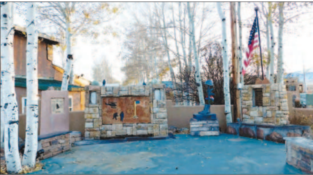
7 Mile Plaza memorial completed
