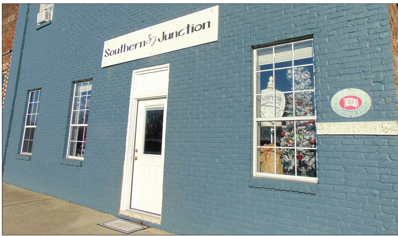
Southern Junction is located in Wartrace's downtown.
