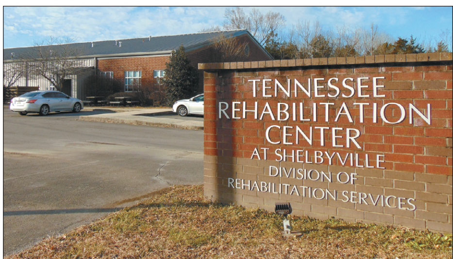
This building on Railroad Avenue will become the new home of Bedford County Emergency Management Agency.
