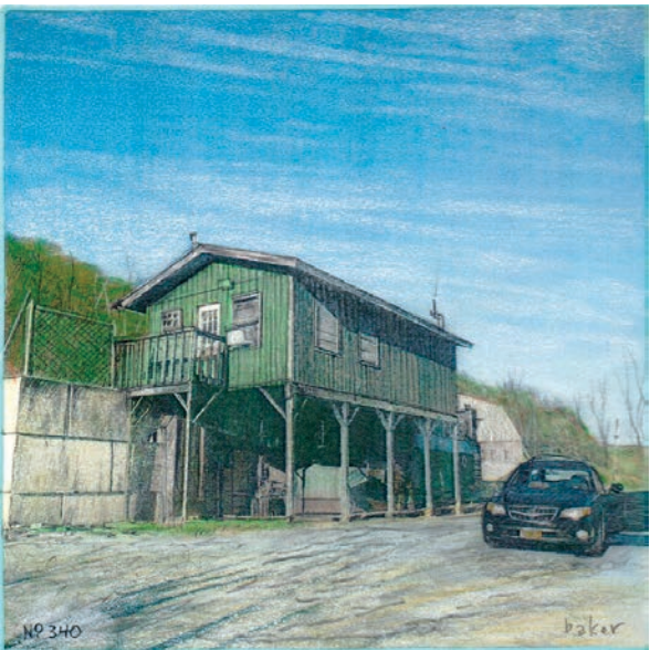
340. Town of Neversink, Transfer Station on Route 55 (06/16/23)
