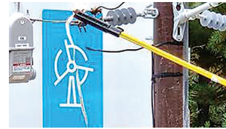
A piece of fabric ribbon completes the circuit between two wires, with potentially lethal results.
