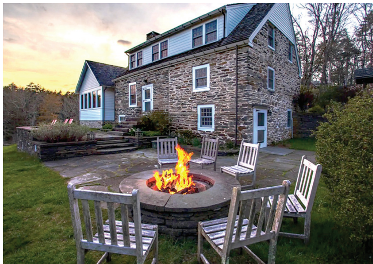
Catskills Concierge offers competitive bids, contract management, and on-site supervision for jobs of all sizes.
