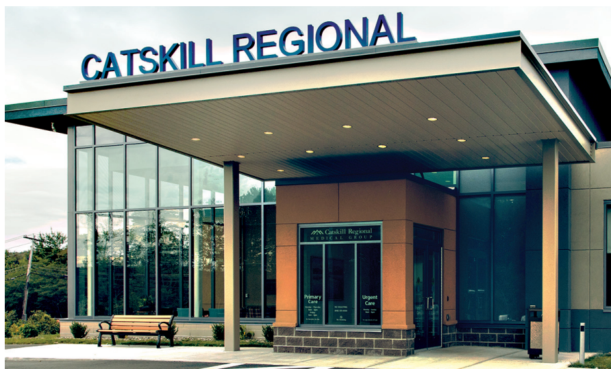
Catskill Regional's Urgent Care building on Concord Rd., Monticello was an Advance Testing project.
