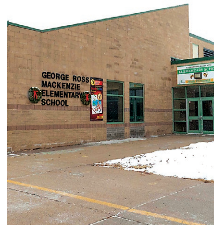
The capital bond project will bring a new roof to the elementary school.
