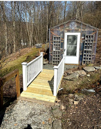
A connecting bridge built by Delaware Handyman and Contracting.
