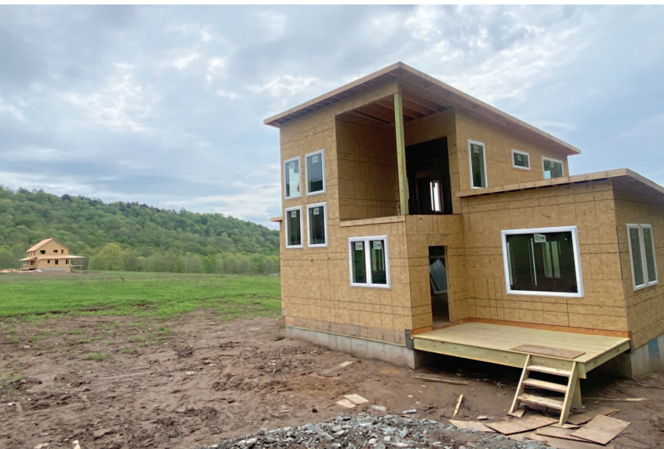
New Construction in Fremont.
