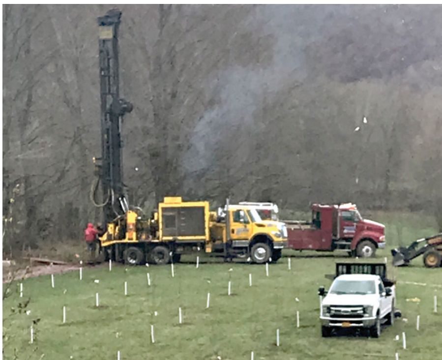
Titan is drilling a well in an apple orchard with a solar pump irrigation system.
