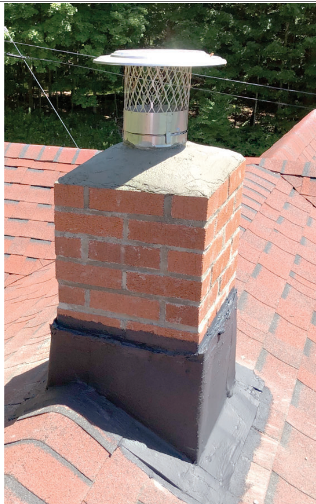
It's important to keep up with chimney repairs.
