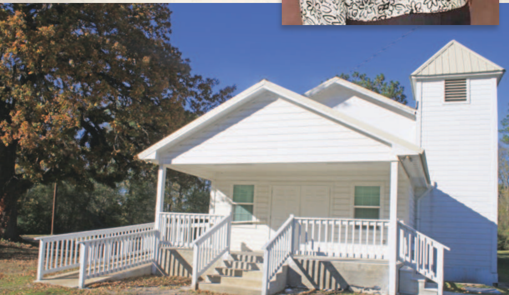
The Ligon Chapel, founded around 1870, remains in use today. Photo by Tony Farkas.
