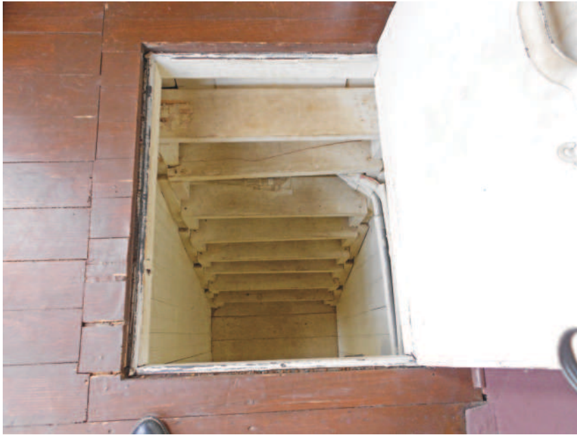
The judge's bench (above) is raised and has a trap door on one side where the judge can escape once the verdict and sentence are rendered. It goes down to an escape route on the first floor (bottom) next to the back door so he can make an escape in the event the decision is unpopular.
