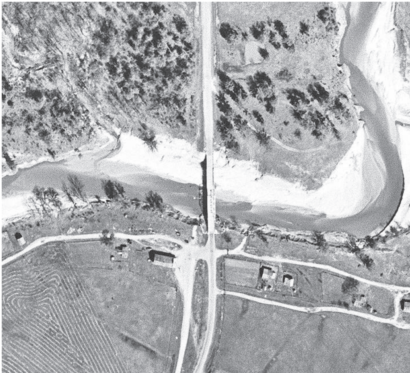
Pictured is Kickapoo Bridge from the 1950s before Lake Livingston was filled.
