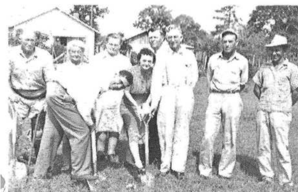
1947 groundbreaking for current church
