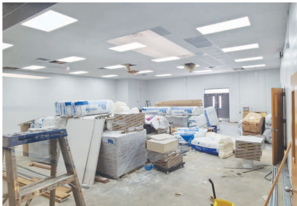
The junior high cafeteria will feature upgrades in plumbing, drainage, cooking and cleaning equipment, serving lines, and undergo an expansion. PHOTO BY BRIAN BESCH
