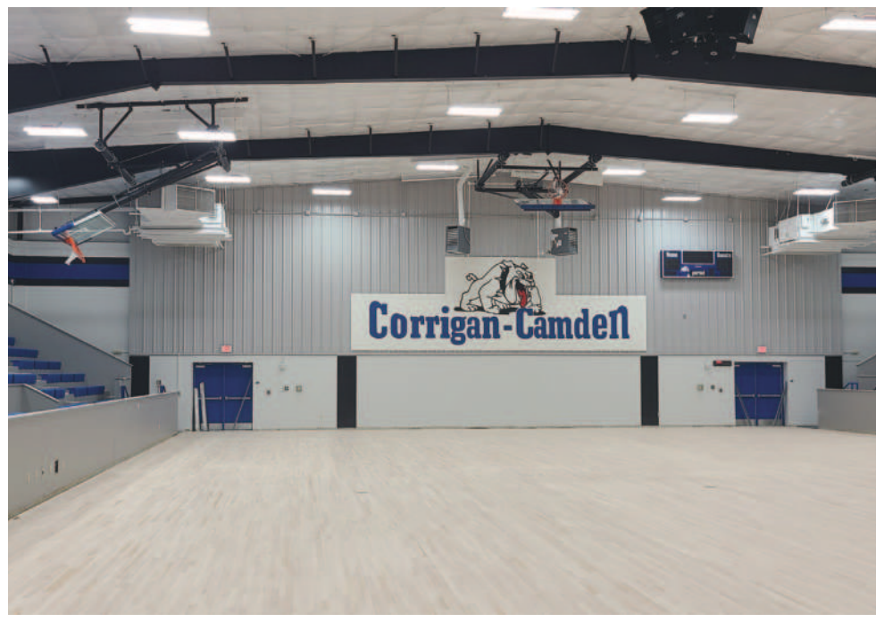
The competition gym is nearly complete, with new paint, floor, seating, and lighting. Under the stands, locker rooms and bathrooms have been renovated. PHOTO BY BRIAN BESCH
