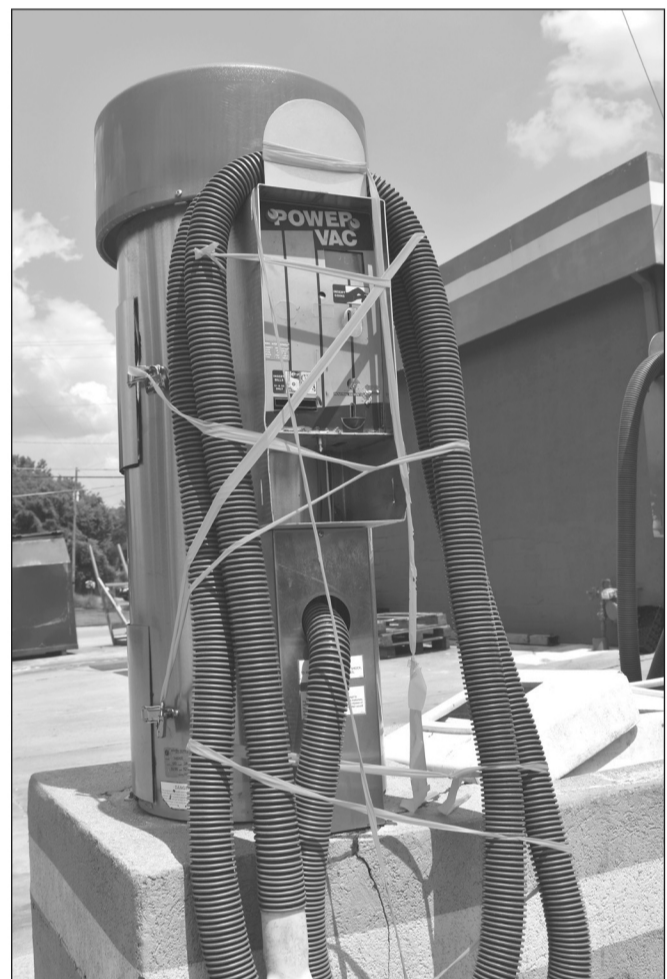
Over $12,000 in damage was done to vacuum machines on July 11. Alexandra Whitbeck / Reporter
