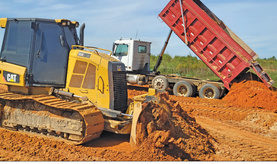
Private contractors assisted in fire efforts by moving dirt.
