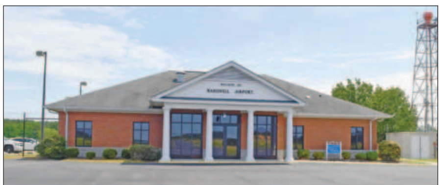
Barnwell Regional Airport terminal offers pilots and passengers a lounge, flight planning room, pilot room with a shower, vending and kitchenette, and Wi-Fi. The terminal is located just minutes away from downtown Barnwell.
