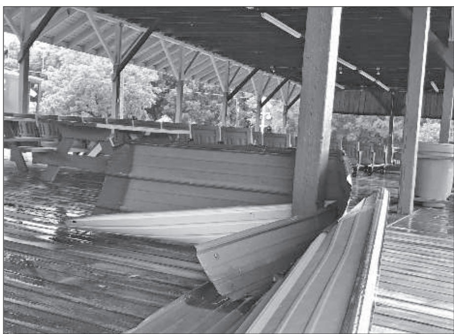
Metal roofing material from a nearby building was blown onto the Hilda Depot.
