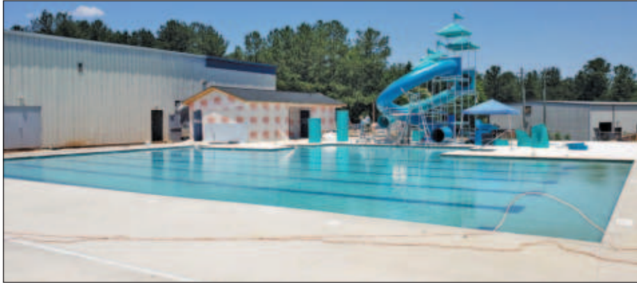
Cool waters will soon draw swimmers to the Barnwell Family YMCA as the aquatics center nears completion.
