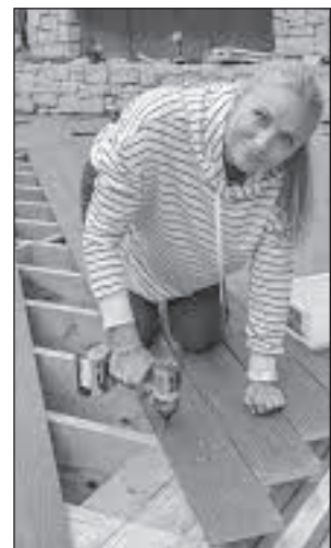
TIVA decking boards are installed on a project.
