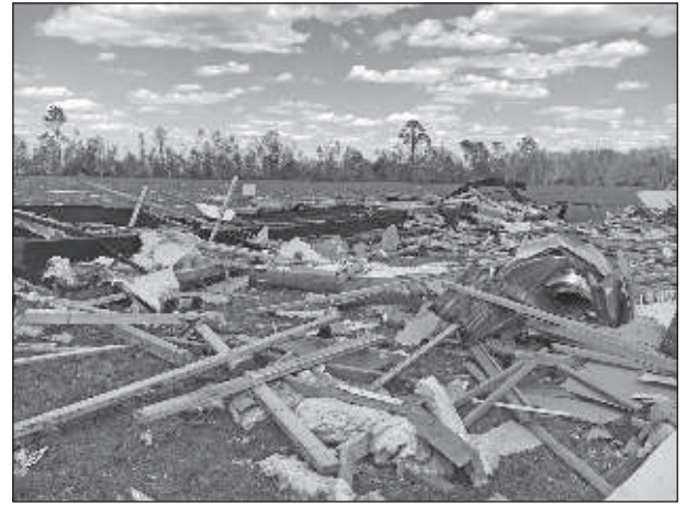
This home on Fitts Road in Allendale was flattened.
