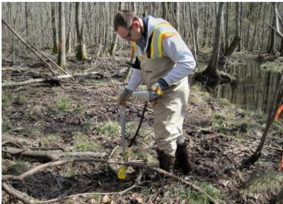
A Savannah River Nuclear Solutions subcontractor technician takes radiological readings of soil near Lower Three Runs, part of a major project to complete the cleanup of a contaminated 25-mile-long stream corridor at the Savannah River Site.
