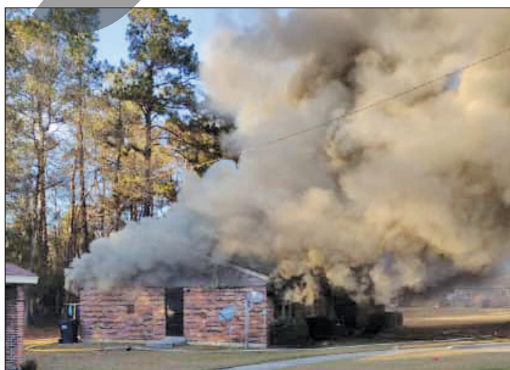
Smoke billows from this duplex at the Lincoln Park Apartments Jan. 17.
