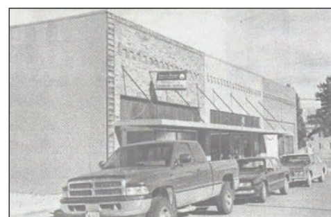
The old Valley Plumbing building will soon be demolished to make way for a new parking lot as part of Torrington's Main Street revitalization district. Photo/Peggy Kerr
