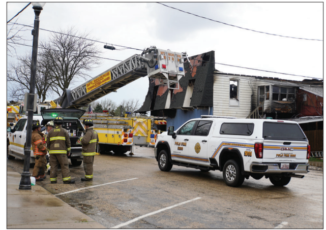
Both 1 and 3 N. Wesley Ave. were made uninhabitable due to the fire. The initial damage estimate to both buildings is $300,000. (Photo by Jeff Helfrich)
