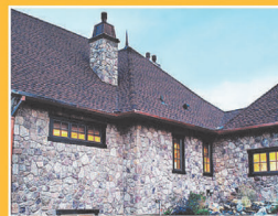
STONE, SIDING & ROOFING
