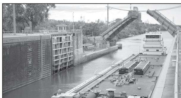
Joliet Lock and Dam
