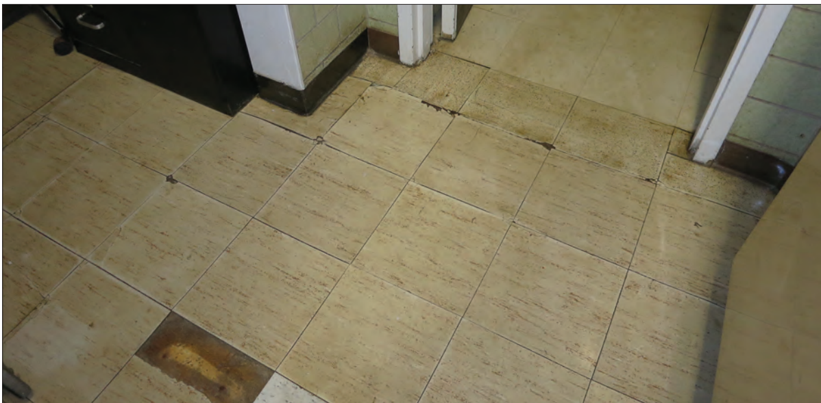
The tours of the junior high were designed to give a full picture of why 272 KIDS is supporting the construction of two additions to the high school and the March ballot referendum that would fund them. Pictured above, is some of the asbestos in the floor tiles that need to be replaced.
