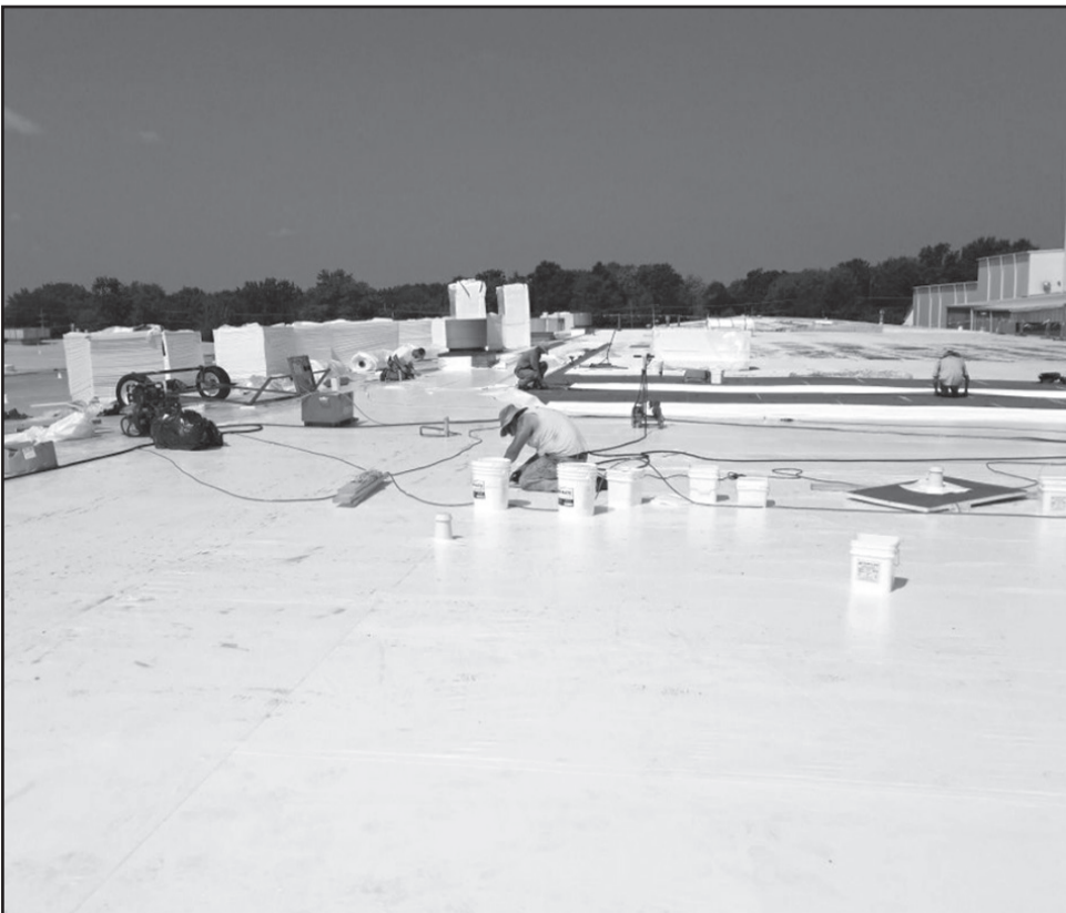
Northern Illinois Seamless Roofing workers install the Duro-Last roofing system on buildings at HCC, Inc., top, and Sullivan's Foods in Mendota, right.
