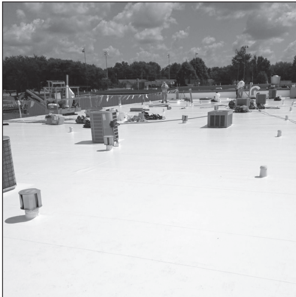
Northern Illinois Seamless Roofing workers install the Duro-Last roofing system on buildings at HCC, Inc., top, and Sullivan's Foods in Mendota, right.
