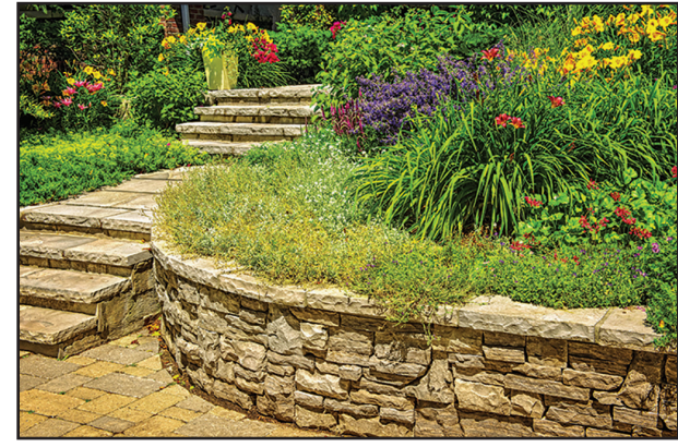
Retaining walls help turn steep slopes in a yard into terraced focal points.
