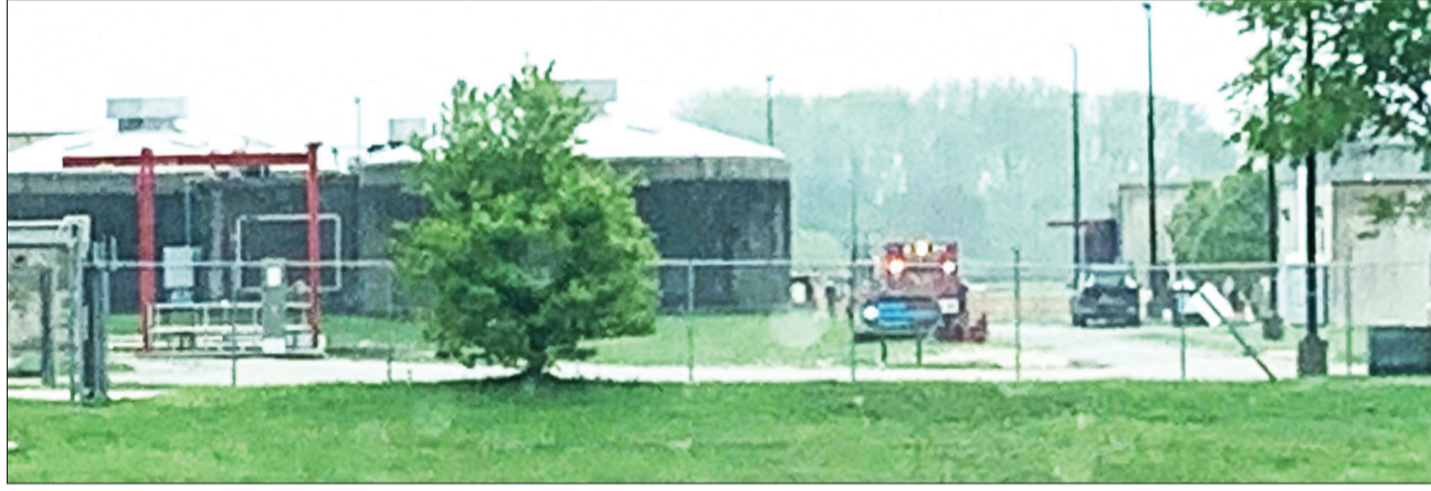
The Rochelle Fire Department responded to the Rochelle wastewater plant Monday morning for a chlorine leak.
