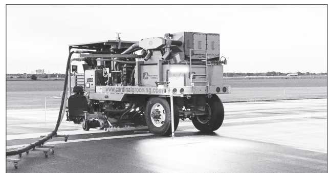
Grooving work being completed on the runway.
