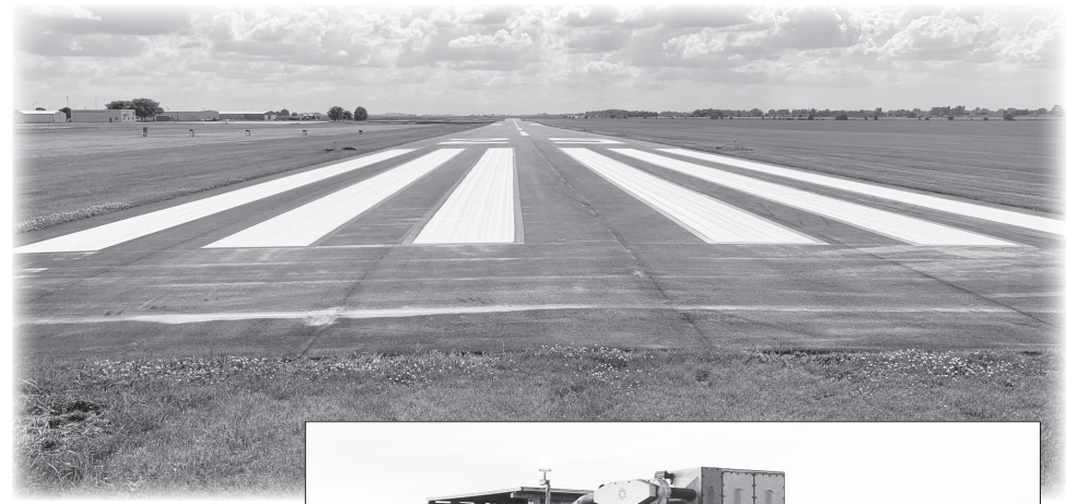
Improvements at Rochelle's Municipal Airport included grooving work on the runway (at right).
