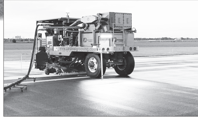
Improvements at Rochelle's Municipal Airport included grooving work on the runway (at right).
